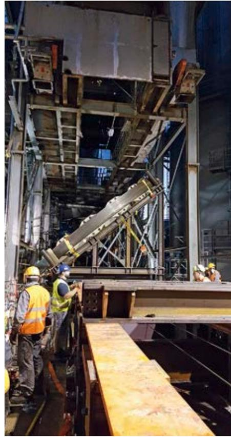
The rear drum ring must first get through the narrow steel construction
