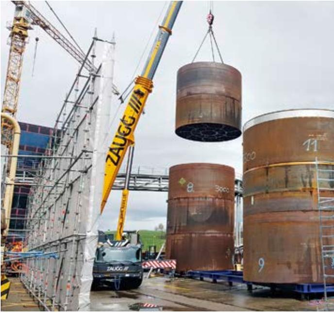
Assembly of the new Büttner drum at the plant directly next to the installation location
