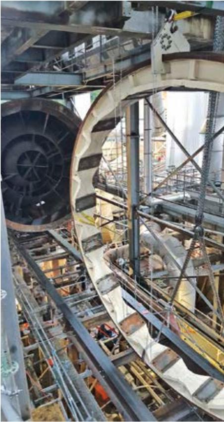
After inserting the drum, the rear drum ring is installed
