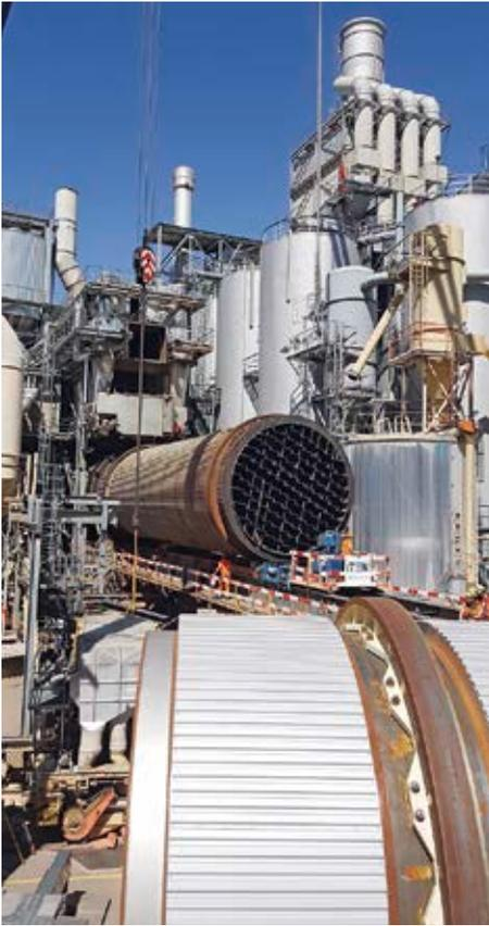
The old drum is moved out, the new drum is ready to be installed
